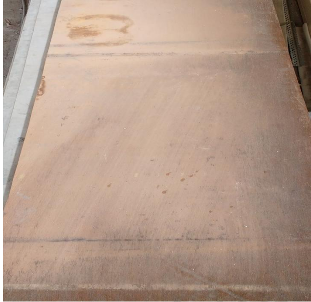
Photograph Exposed face before starting the test
